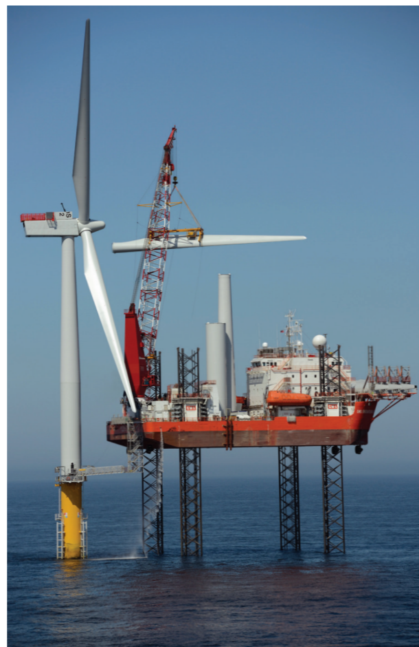
Different phases of turbine installation including lifting the nacelle on to the tower (top left) and installing blades (above and right).
